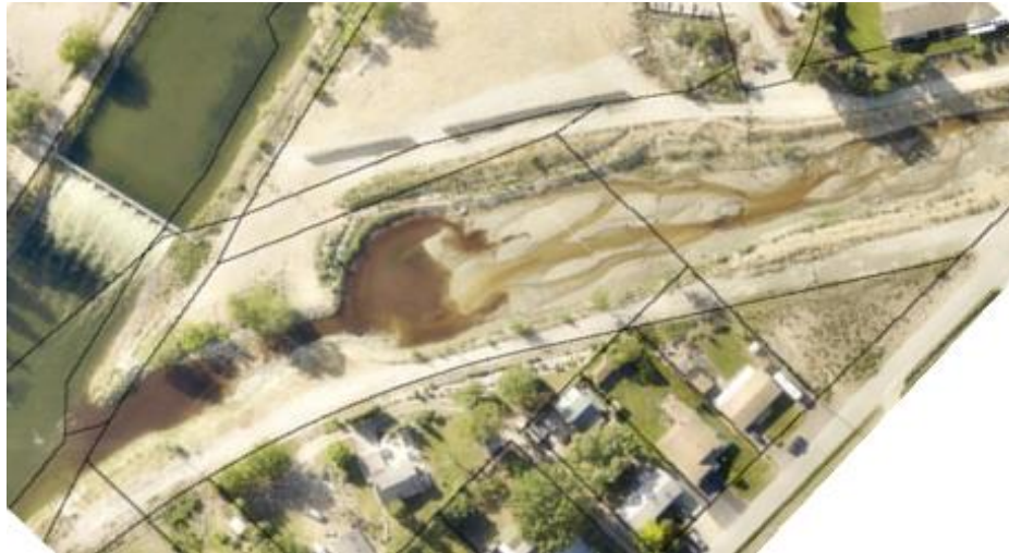
Figure 4. Sediment trap at the mouth of Shuttleworth Creek near its confluence with the Okanagan River.
