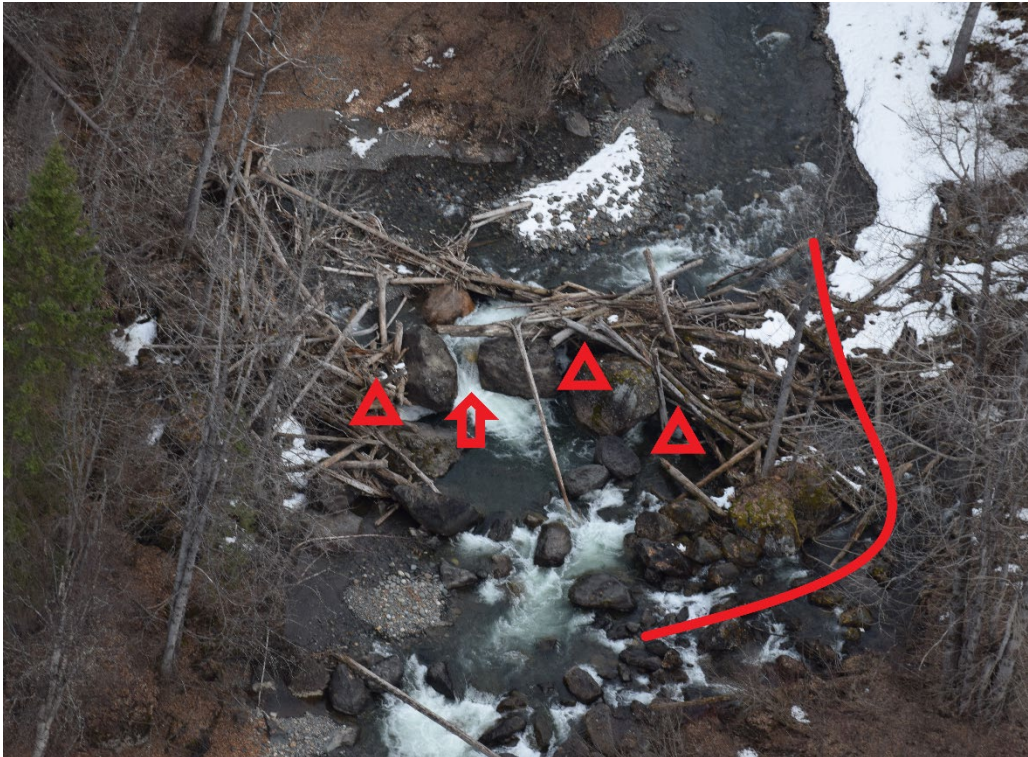
Photo 1: The debris jam on King Salmon Creek, April 21 st , 2019. The triangles mark the location of potential historic spill points, the red arrow is the only currently passable spill point and the red line is a historic by-pass channel.
