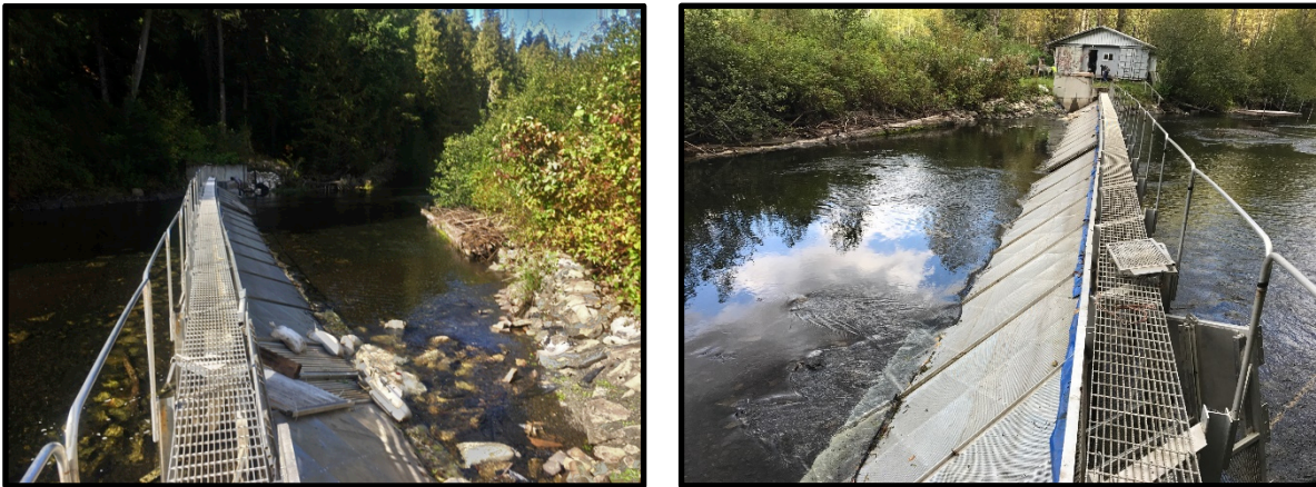
Figure 5: KsF on September 11 th , 2017 after set-up.
