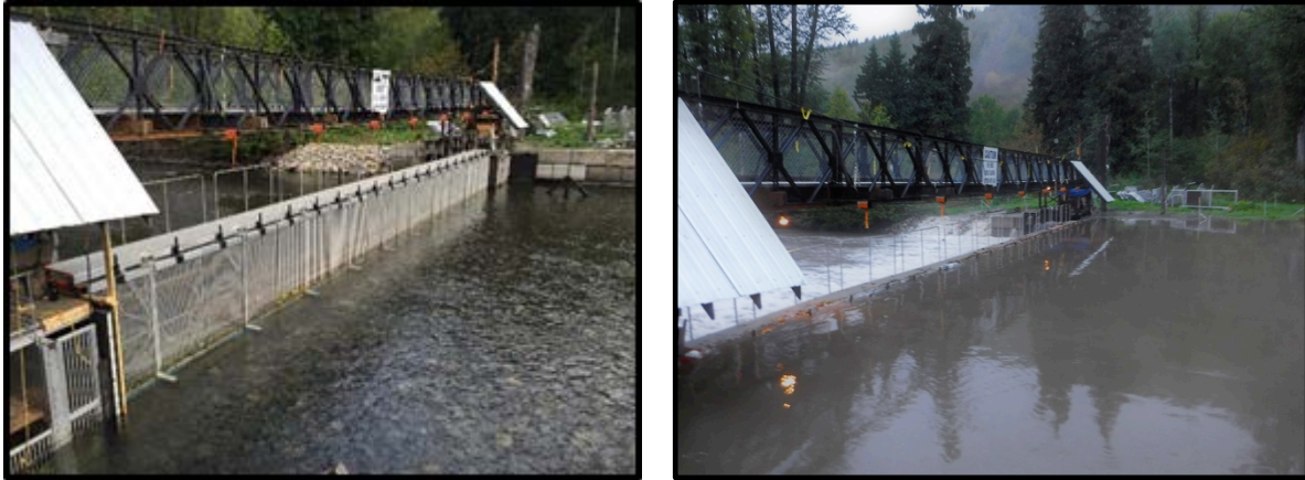
Figure 4: Photo on left - taken during normal operating flow and photo on right on September 11 th , 2017, during extremely high flow.
