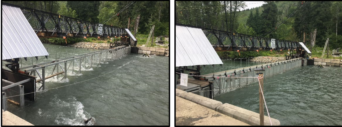
Figure 2: Photo series of installation of the KSEF structure.
