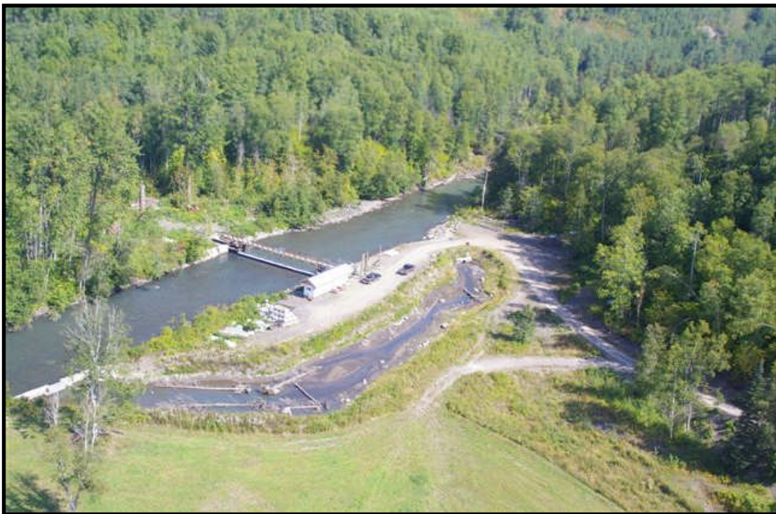
Photograph 1. Aerial view of the Kitwanga River Salmon Enumeration Facility.
