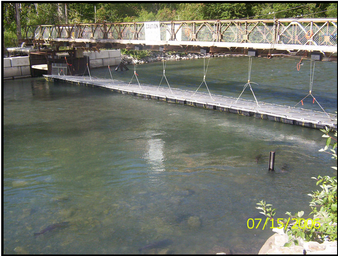
Photograph 2. Floating panels attached to overhead walkway bridge.
