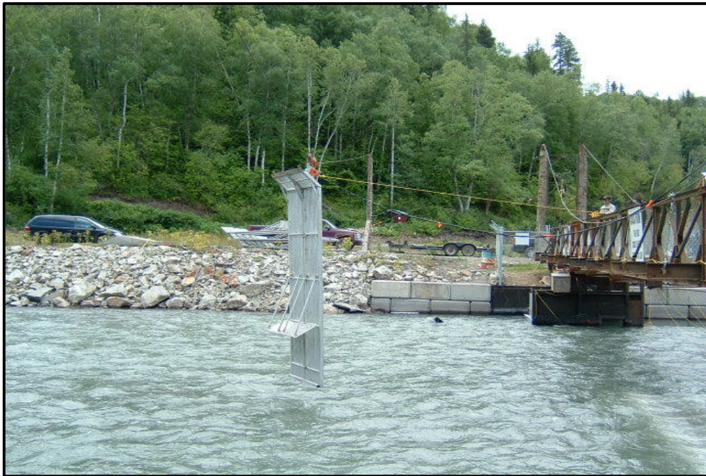
Photograph 3. Overhead winch used to lower aluminium panels into river
