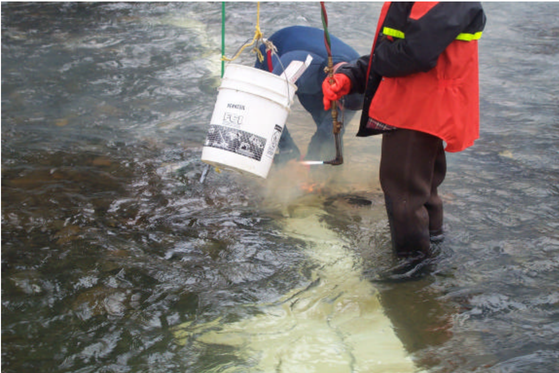
Photograph #9: Cutwaters being cutout to allow for proper fence panel installation.
