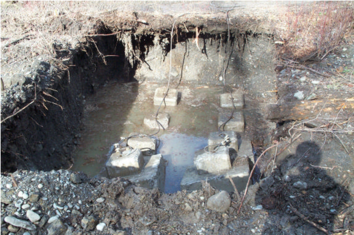
Photograph #7: Installation of "A" frame anchors.
