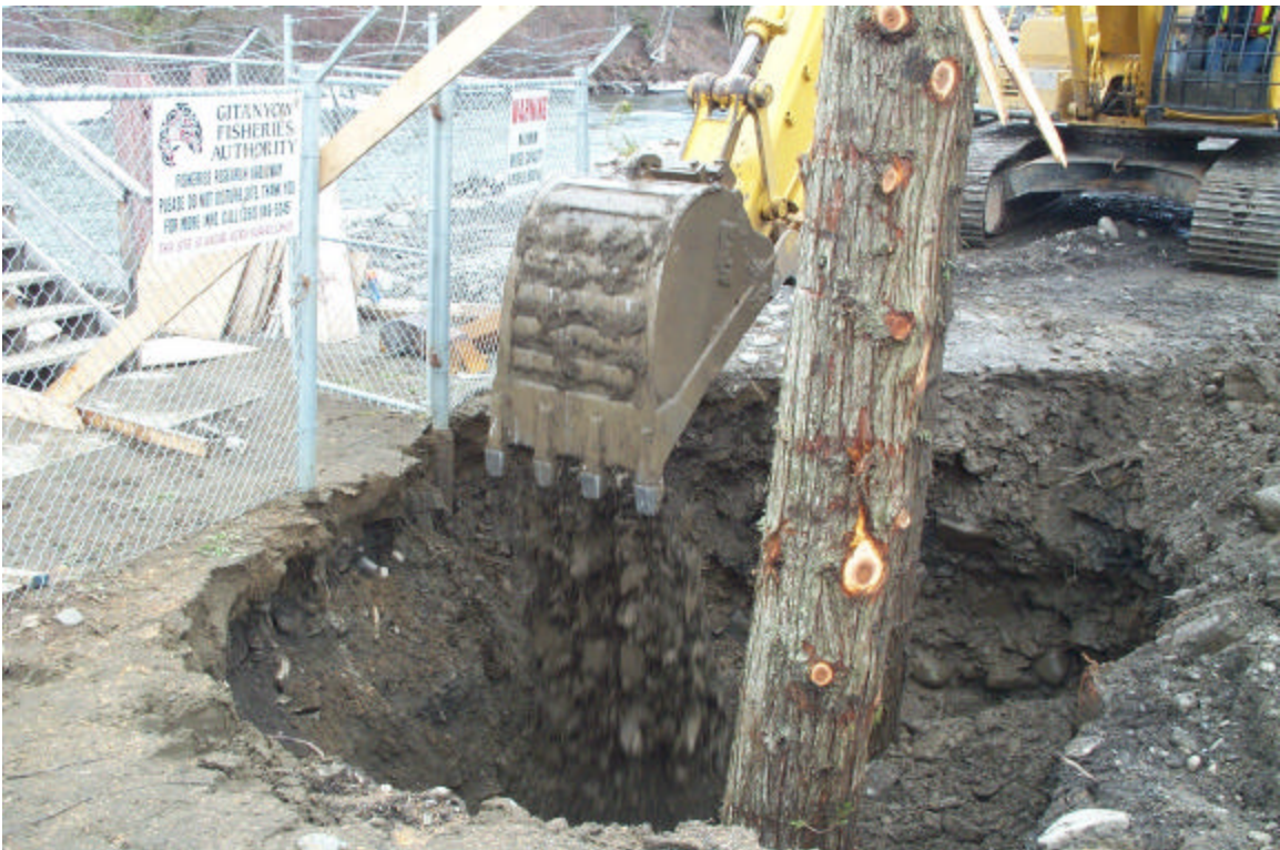
Photograph #5: "A" frame installation.
