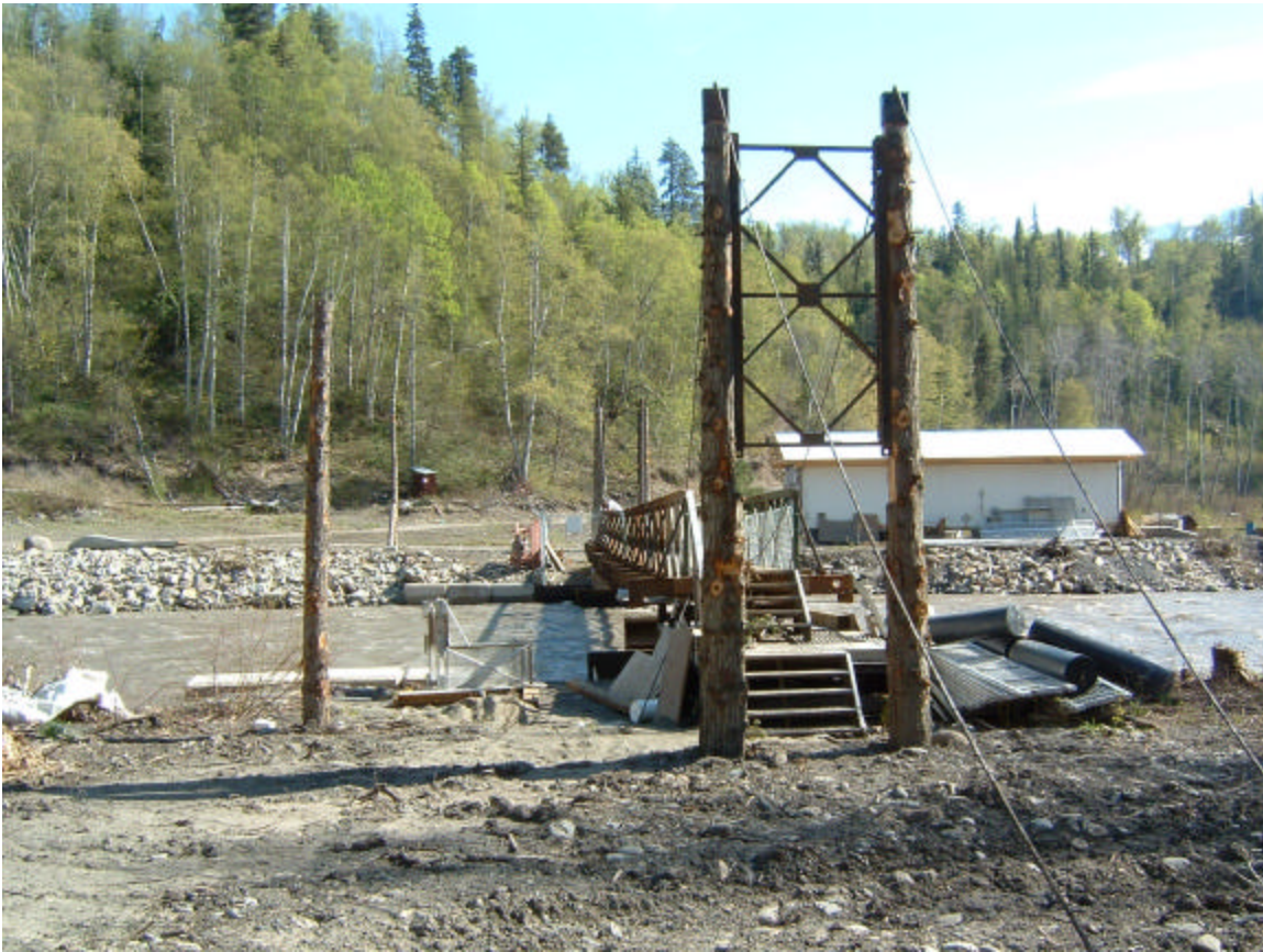
Photograph #8: Completed "A" frames and re-enforcement cables.
