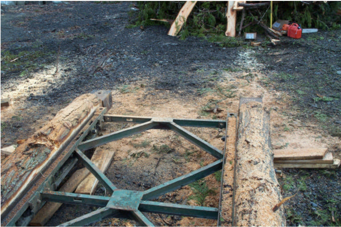
Photograph #4: "A" frame construction.
