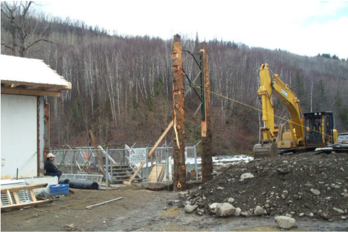
Photograph #6: Installed "A" frame.
