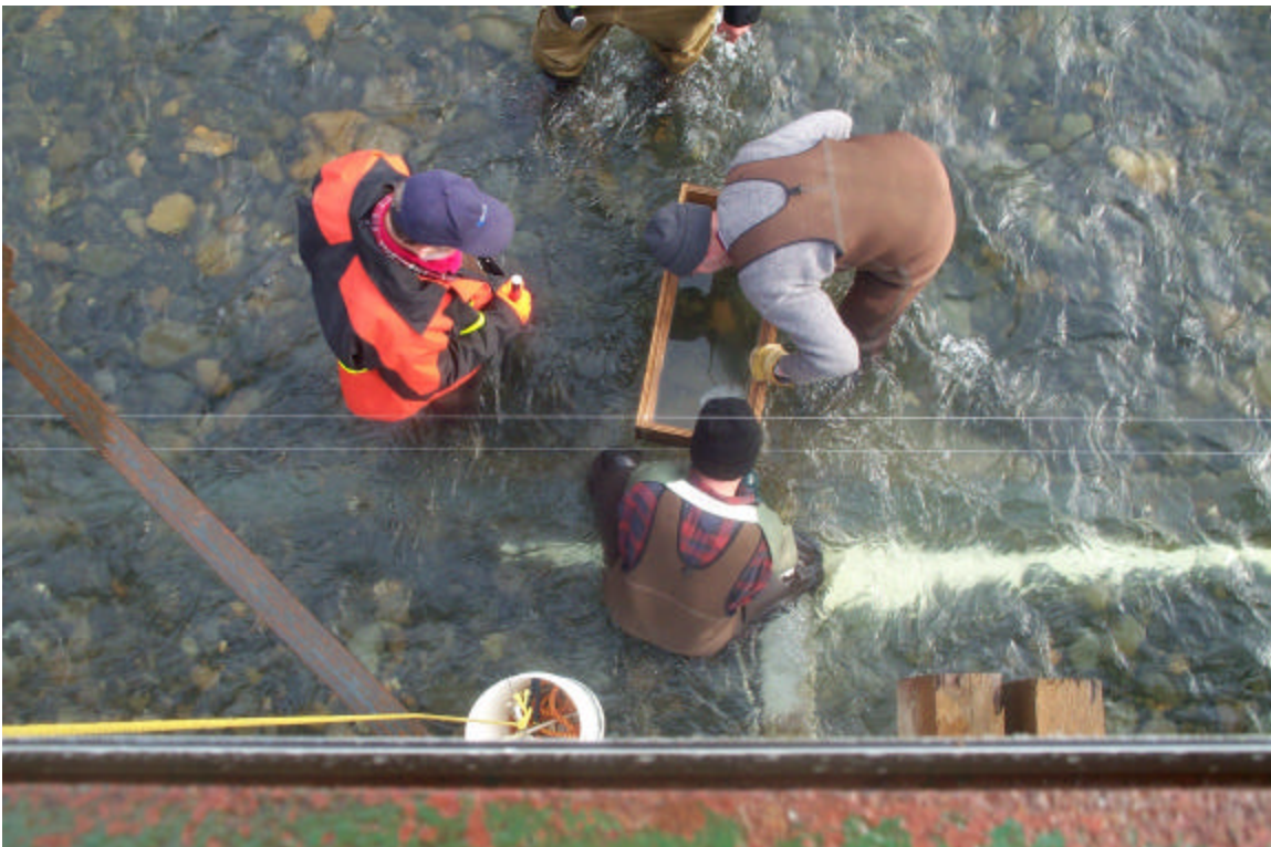
Photograph #2: Fence hooking bracket installation.
