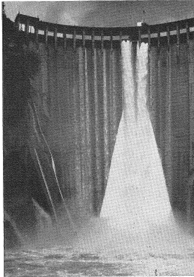
FIGURE 17. Flow over the spillway at Baker Dam with one gate fully open and adjacent gates cracked one foot.
