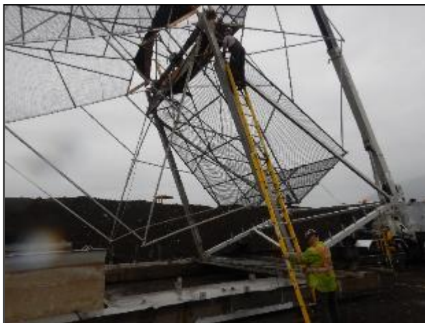
Raising the baskets and attaching the axle to the tower assembly.
