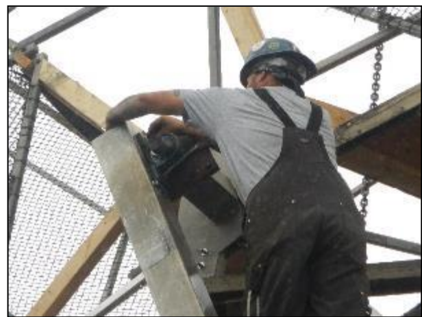
Raising the baskets and attaching the axle to the tower assembly.
