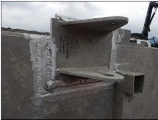
Pictures of tower pivot and pontoon repairs and re-enforcements.
