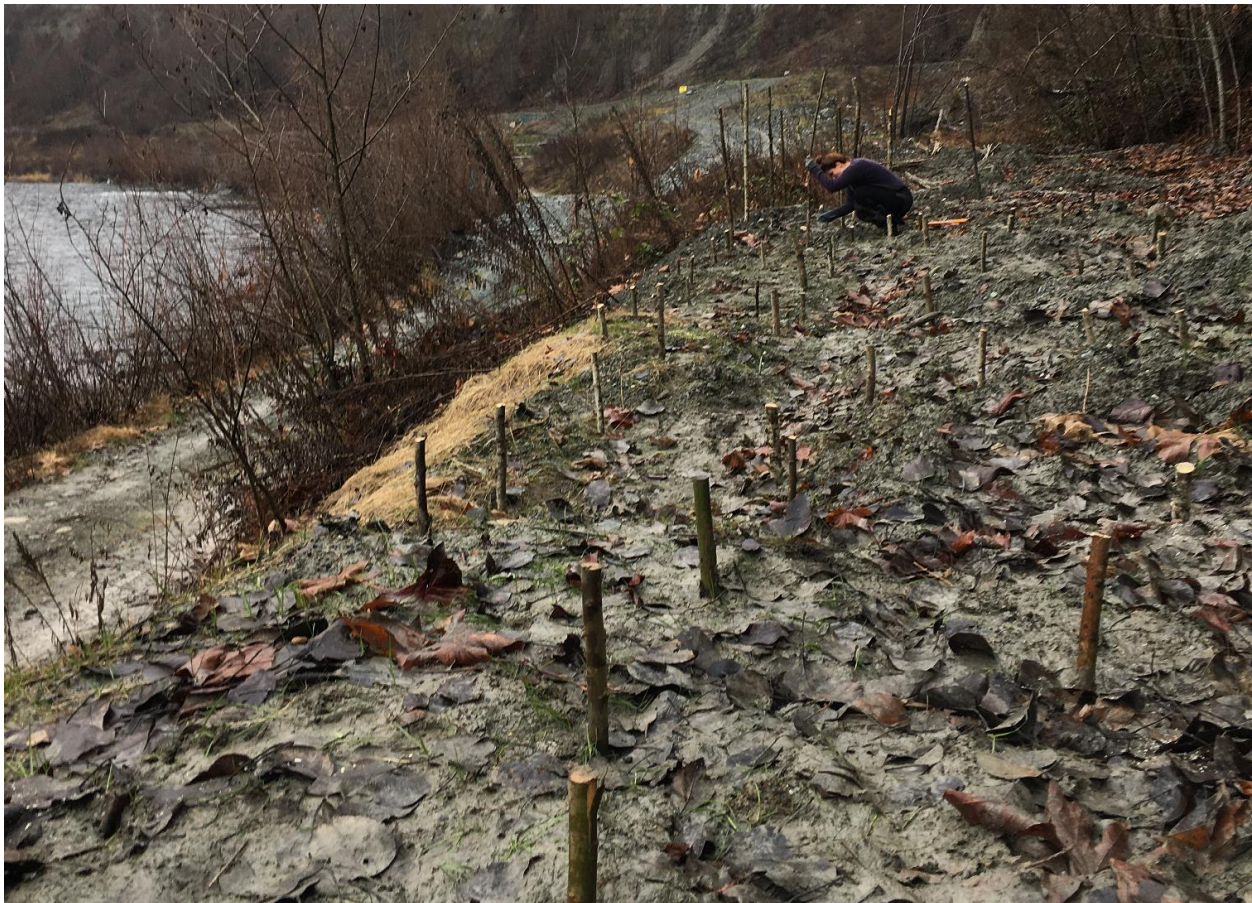
Figure 3. Bioengineering work completed at Stoltz Bluff during the winter of 2019/20.
