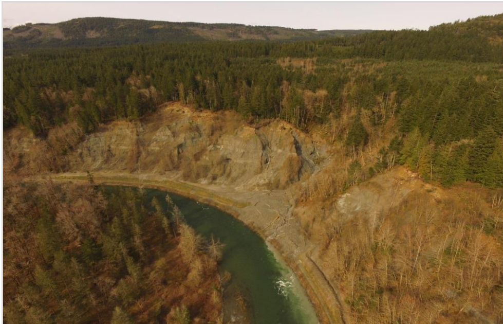
Figure 2. Aerial view of Stoltz Bluff following the Clearwater Creek slope failure in 2017. The sediment flowing from the creek into the Cowichan River can be seen on the center-right of the photo, as can damage to the access road.
