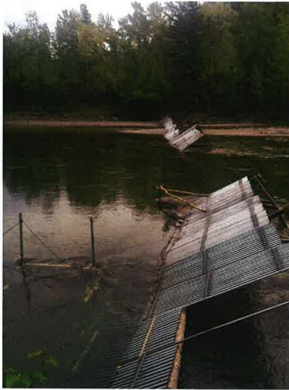
Photograph 1. 2018 Sonar and partial fence, note low water levels.
