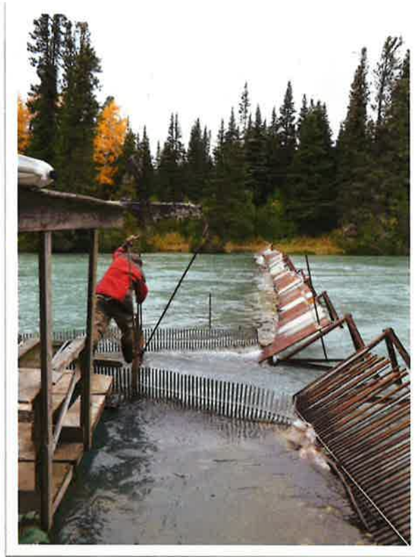
Photograph 1. Little Trapper Lake Weir.
