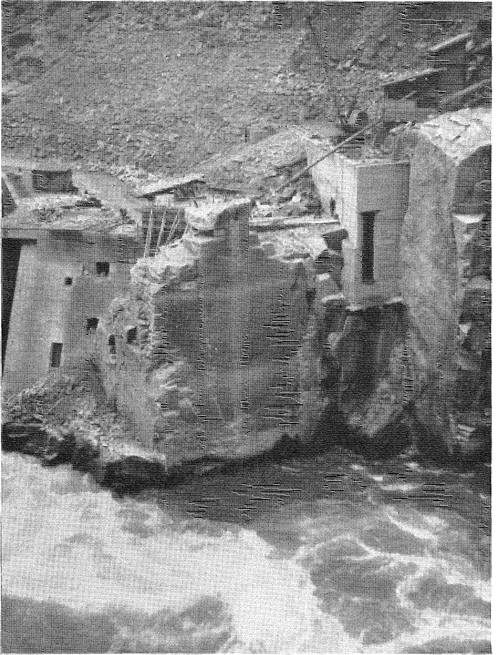
FIG. 1—The high level fishway at Hell's Gate, finished in 1951, to facilitate passage of early runs such as those destined for the Stuart, Bowron and Nadina Rivers. This fishway will begin operating as the lower level fishway becomes flooded by rising water.
