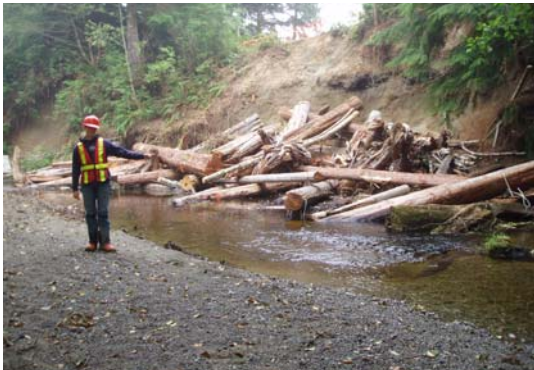
Figure 3. Site LS2-1 after restoration.
