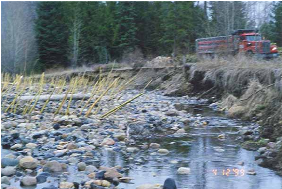
Figure 27: Willows stakes were planted in this gravel bar during the winter of 1999 on Besette Creek to help stabilize the bar and to eventually concentrate the high flow to the other (left) side of the creek.
