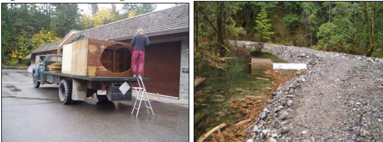
Figure 4 Beaver boxes being constructed and after installation
