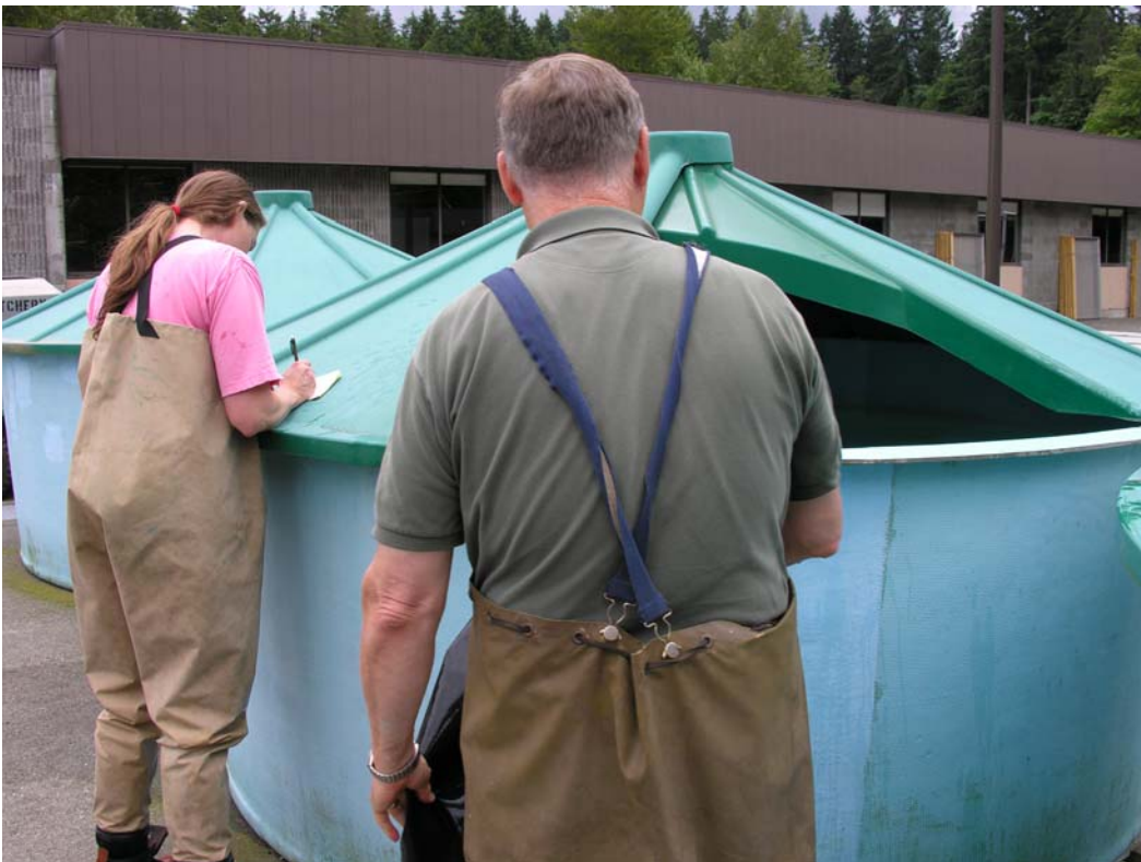
Figure 28. 10-ft diameter fish holding tanks at Puntledge Lower Site.
