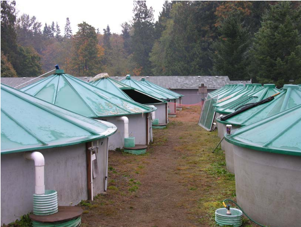
Figure 40. 20-ft diameter holding tanks (5 tanks on the left) at Rosewall Creek hatchery.
