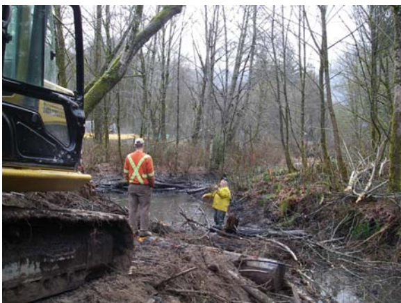
Figure 2 – Deepening of the Britannia Tidal Slough
