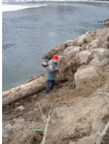
Hand planting of Willows and Aspen on Toe.
