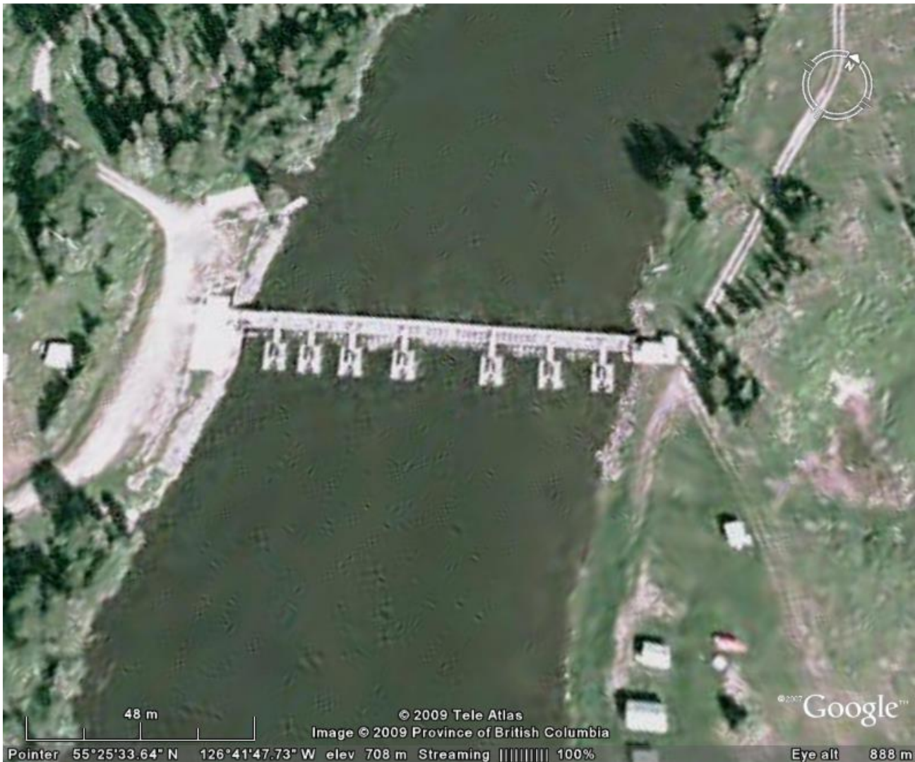
Appendix A. Aerial view of the Babine river counting fence. Traps 1-3 are on the right hand side. The building used to store the batteries and recording equipment is on the right hand abutment.
