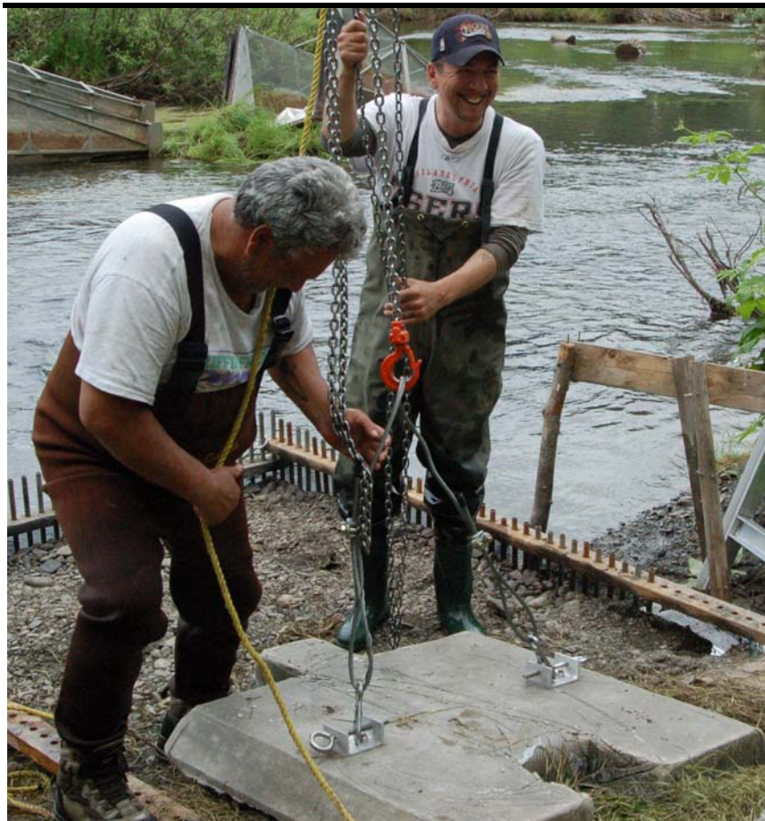
Figure 3. Concrete block being moved into position.
