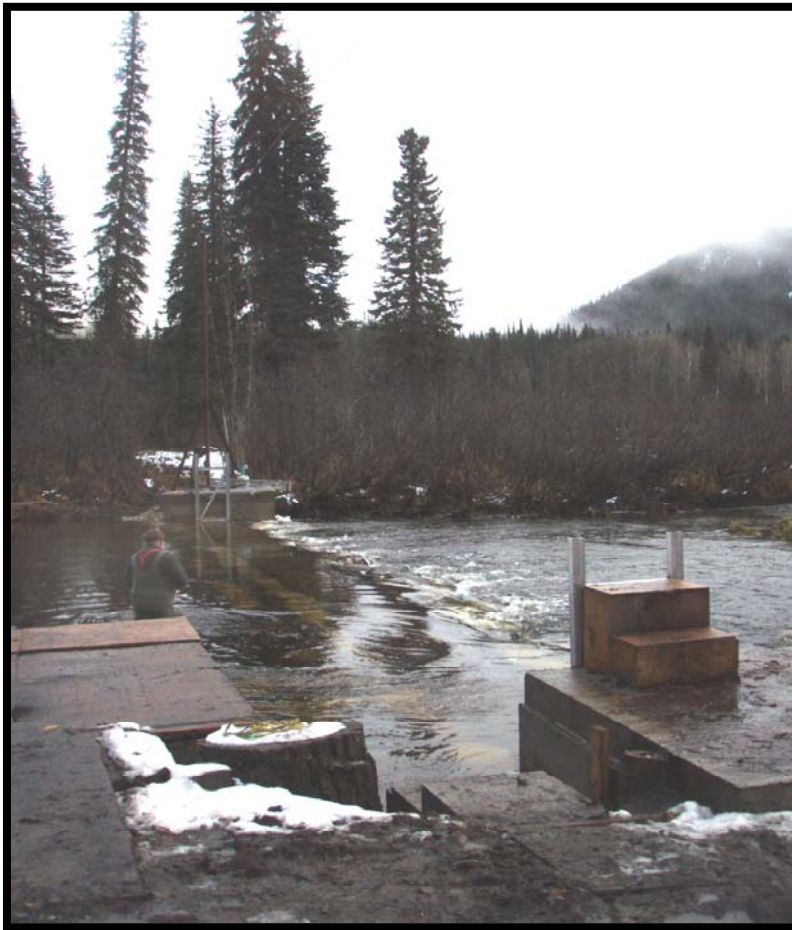
Figure 8. Cement piers at each bank anchor the weir in place.
