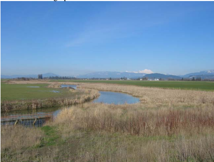
Photo 2. Looking upstream of Tide Gate
