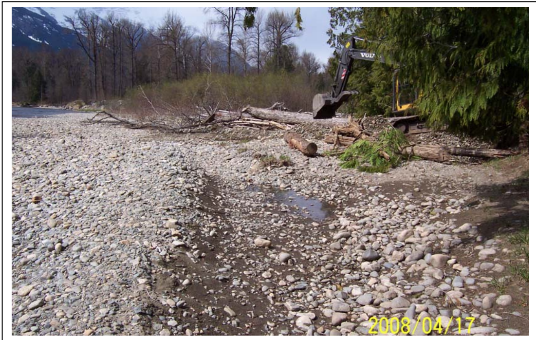
Figure 2. Intake channel befor construction
