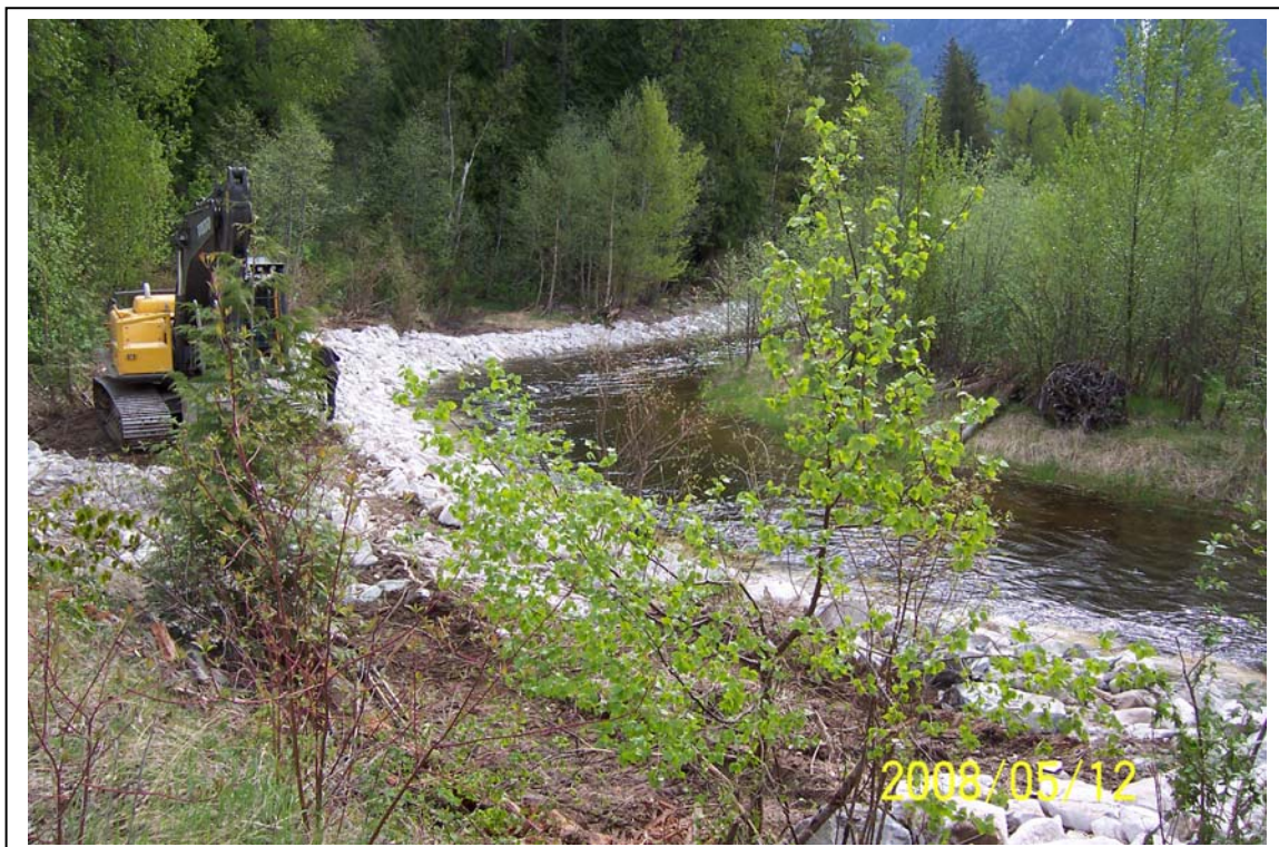
Figure 5. Intake channel with bank armor.
