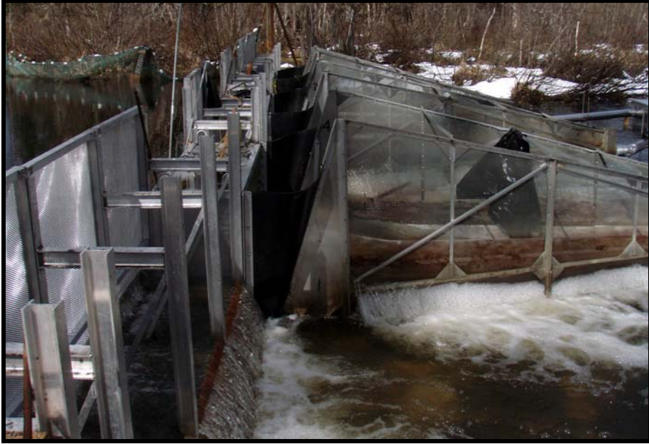
Figure 1. Fence structure shows screens in upstream position and traps mounted with adaptors.
