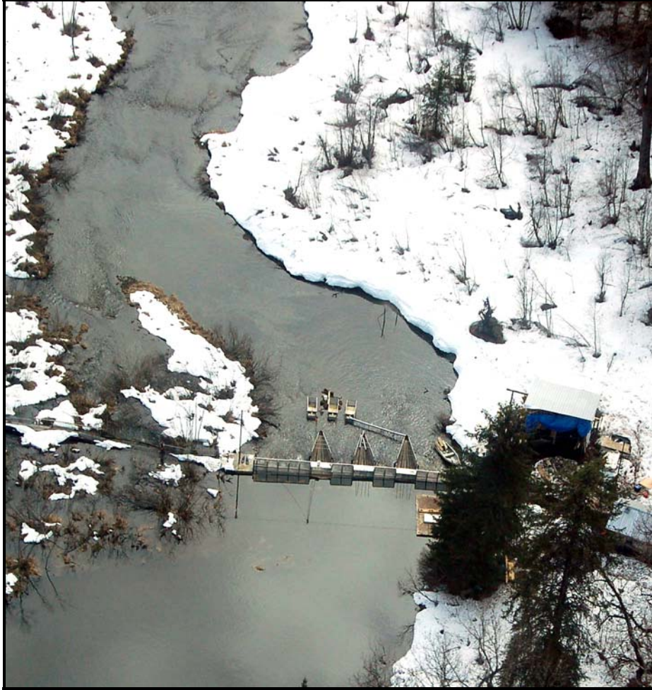
Figure 2. Three fan traps in position mounted in the Slamgeesh Weir.
