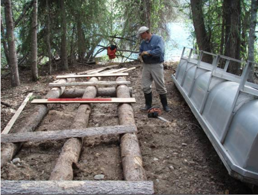
Figure 3. Preparation of site and bases for Capilano troughs.
