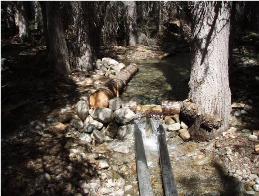
Figure 4. Dam and water impoundment structure.
