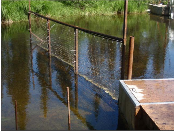
Figure 7. Steel welded frame weed catcher upstream of smolt trap location.
