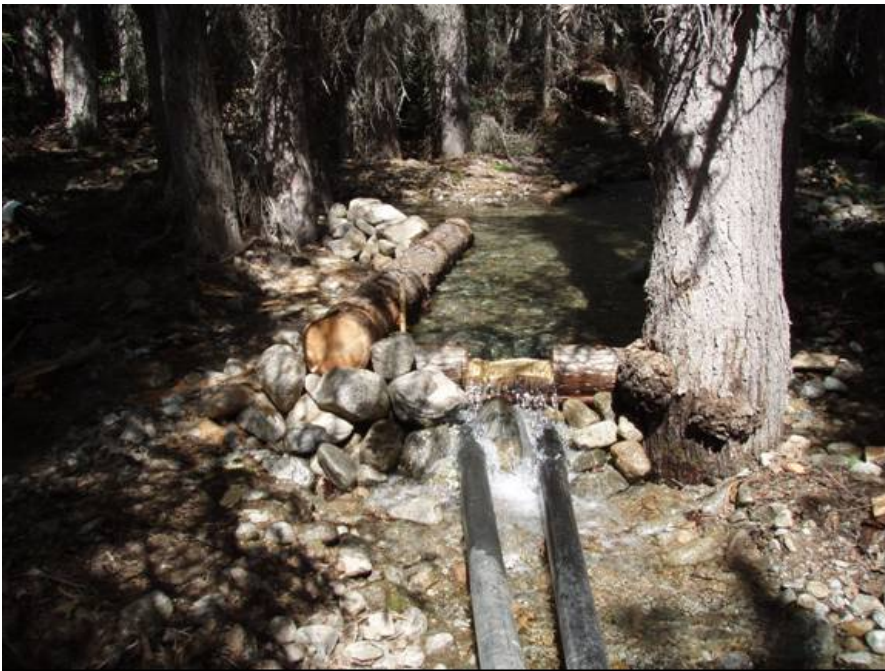
Figure 2. Dam and water impoundment structure.
