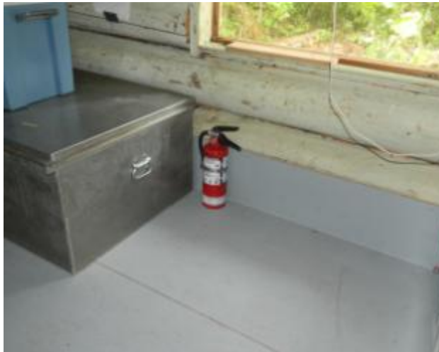
Figure 8. A section of the new floor in the main cabin at Slamgeesh camp in July 2012.
