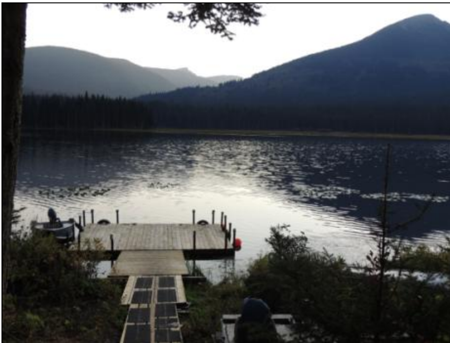
Figure 7. The newly completed dock at Slamegeesh camp in July 2012 prior to attachment of fender floats.
