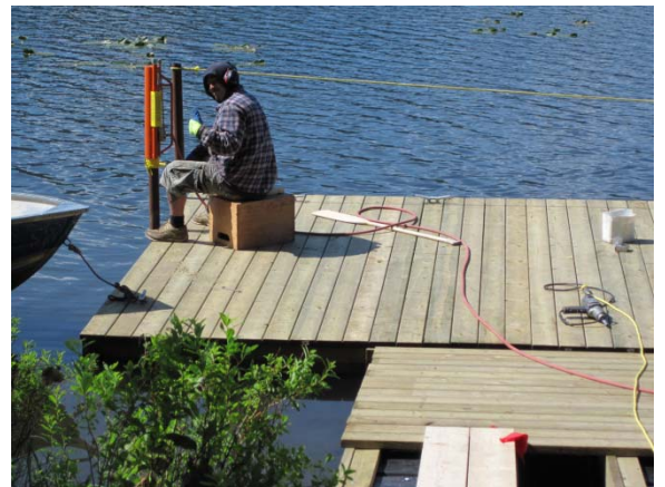
Figure 4. Instalation of drill pipe protection around dock.
