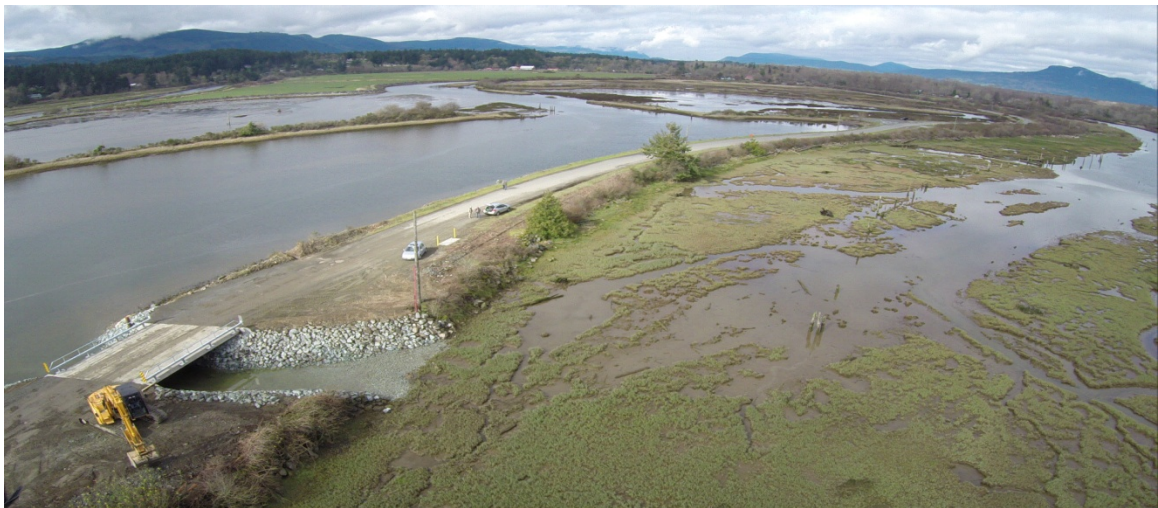
The new bridge across the Causeway that splits the Cowichan Estuary in half.
