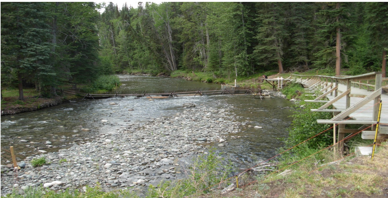
Appendix C- 2. Little Tahltan River weir, 2014.
