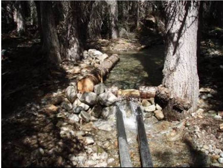
Figure 2. Dam and water impoundment structure.
