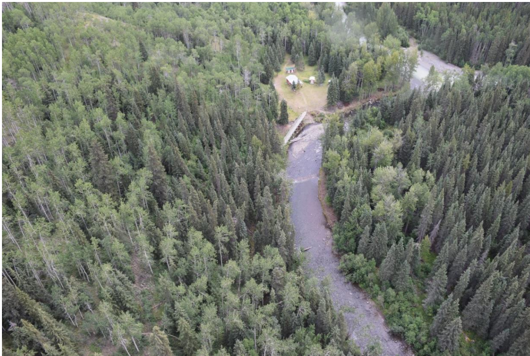
Photo 2: Aerial view of Reach 1 on the alluvial fan.
