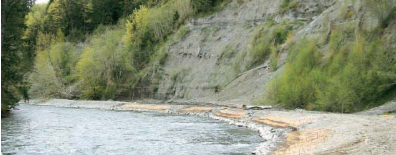
Stoltz Slide Remediation - After
