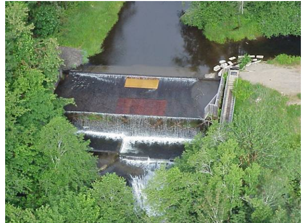
Goldsborough Dam Before Removal
