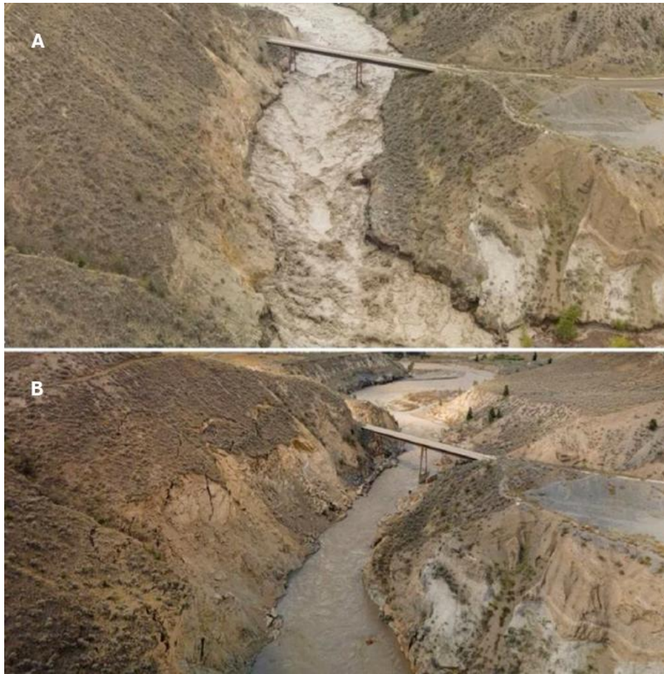
Figure 9. Farwell Canyon A) during the outbreak flood, and B) as waters rescinded and left massive tension cracks in the rock hillside (to the left).
